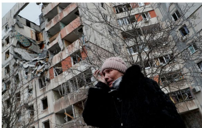
An apartment block in Mariupol, destroyed by Russian shelling | CREDIT: ALEXANDER ERMOCHENKO / REUTERS
